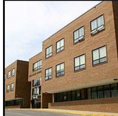
Pictured from top to bottom: Sligo Creek Elem. School; East Silver Spring Elementary School; Portable passageway at Takoma Park Elementary School; Piney Branch Elementary School.
