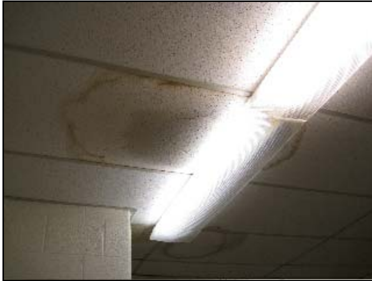
Room C123-Ceiling has bulging wet tiles. 1
