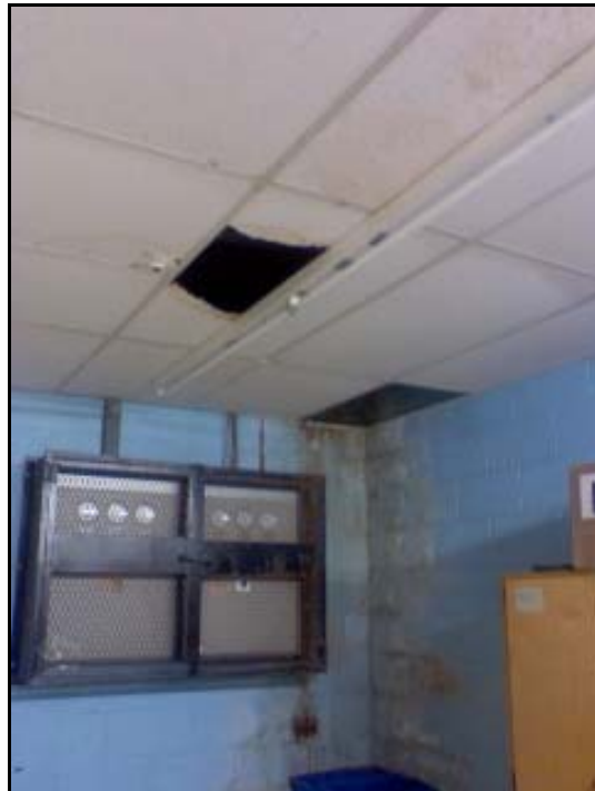
Room C123-Ceiling has bulging wet tiles. 1
